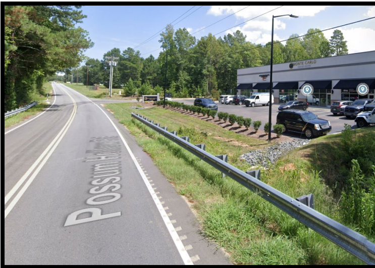
Looking East along Possum Hollow Road
