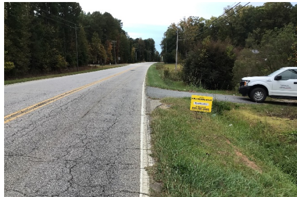
Looking south along Monroe Highway with subject parcel to the right
