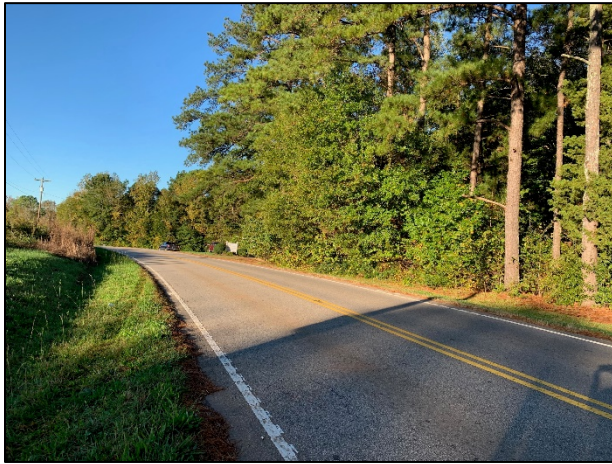
Looking west along Shelley Mullis Road
