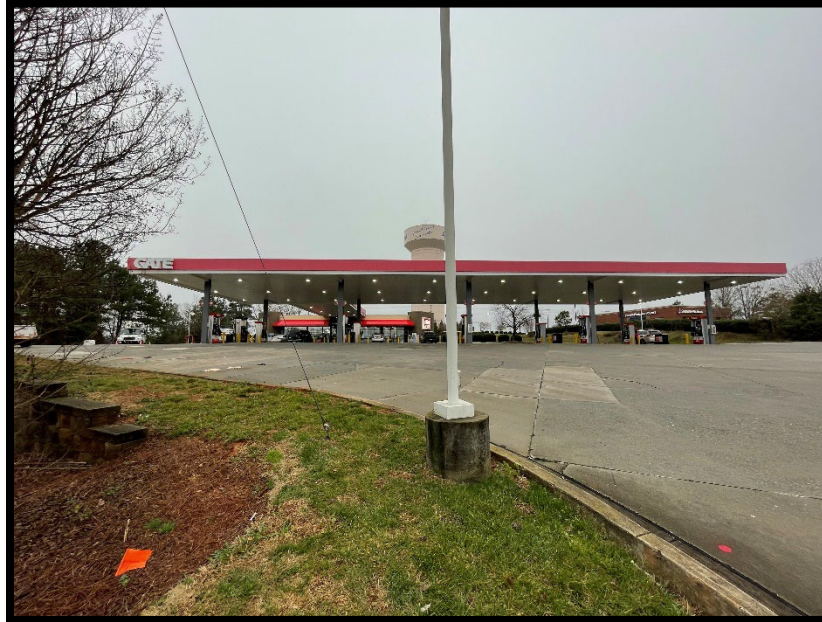
Facing the Gate Station
