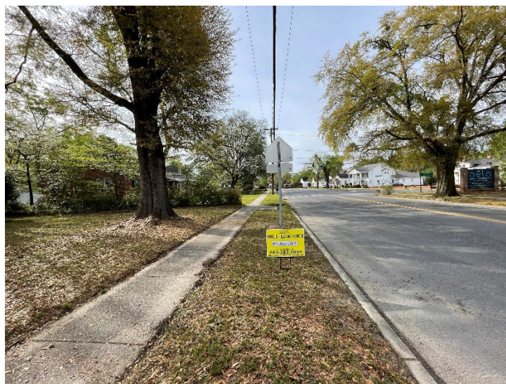
Facing South on North Matson Street
