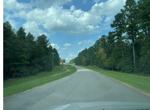
Catawba Ridge Boulevard facing north at Proposed Access “A”
