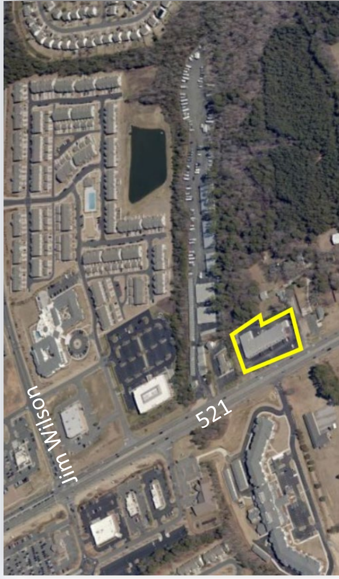
Aerial view looking north on Hwy 521: Subject parcel can be seen outlined in yellow
