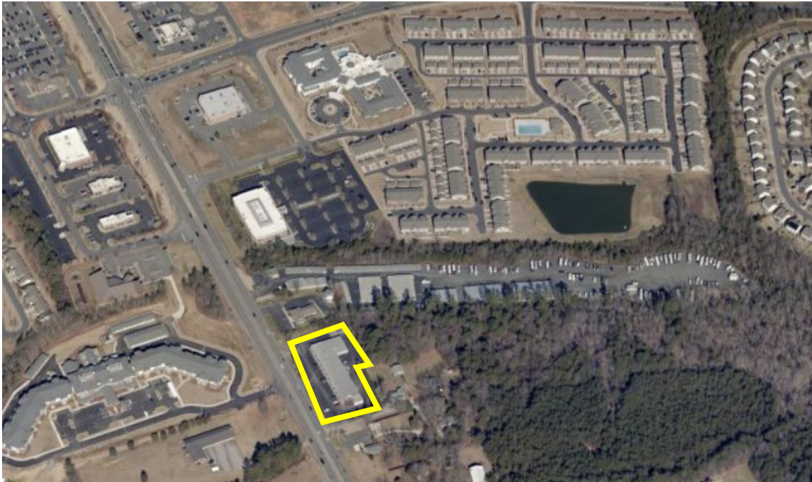
Aerial view looking north on Hwy 521: Subject parcel can be seen outlined in yellow.
