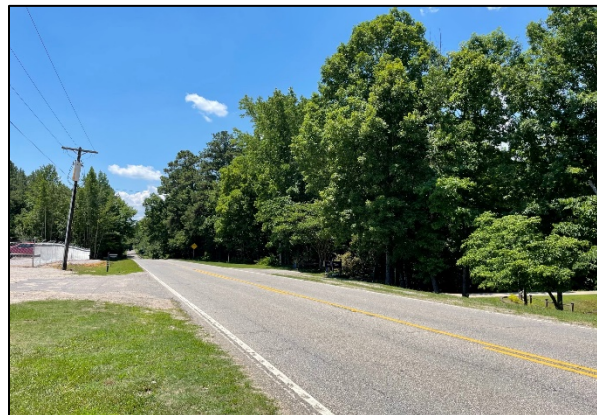
Looking south along Kershaw Camden Highway
