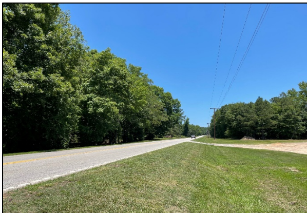
Looking north along Kershaw Camden Highway
