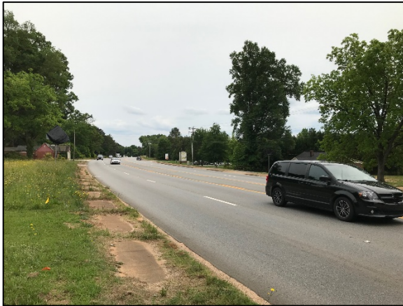
Looking south along US-521
