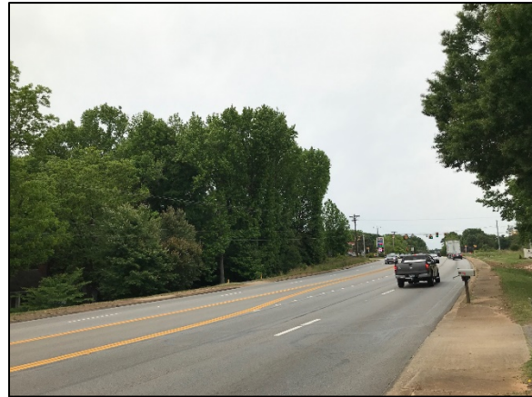
Looking north along US-521
