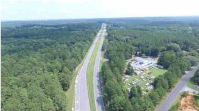
US 521 at East Rebound Road, view North
