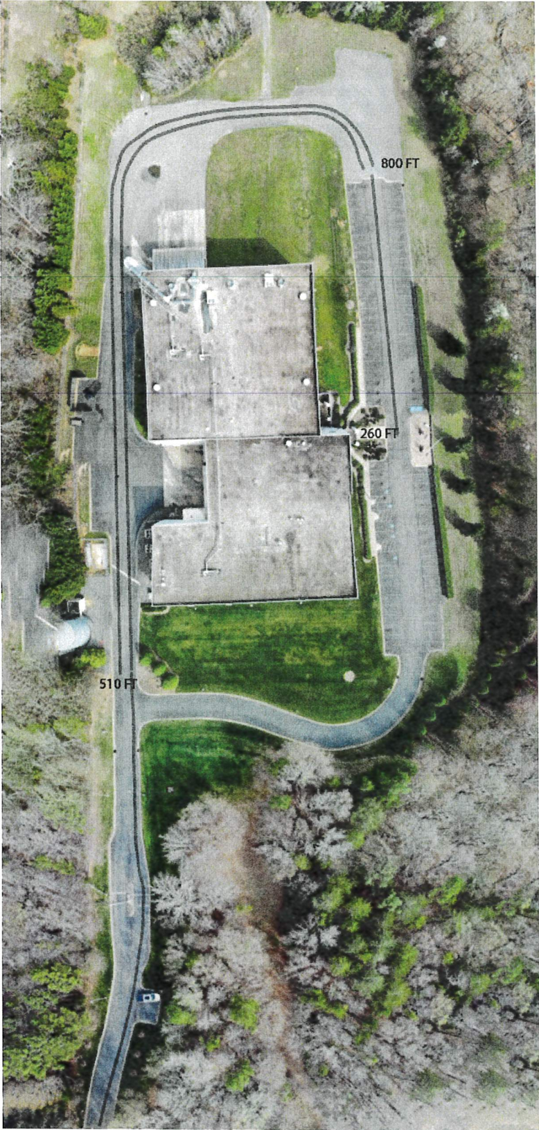
Aerial Photograph of the Building Footprint for Traffic
