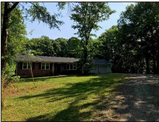
Looking directly at one subject property
