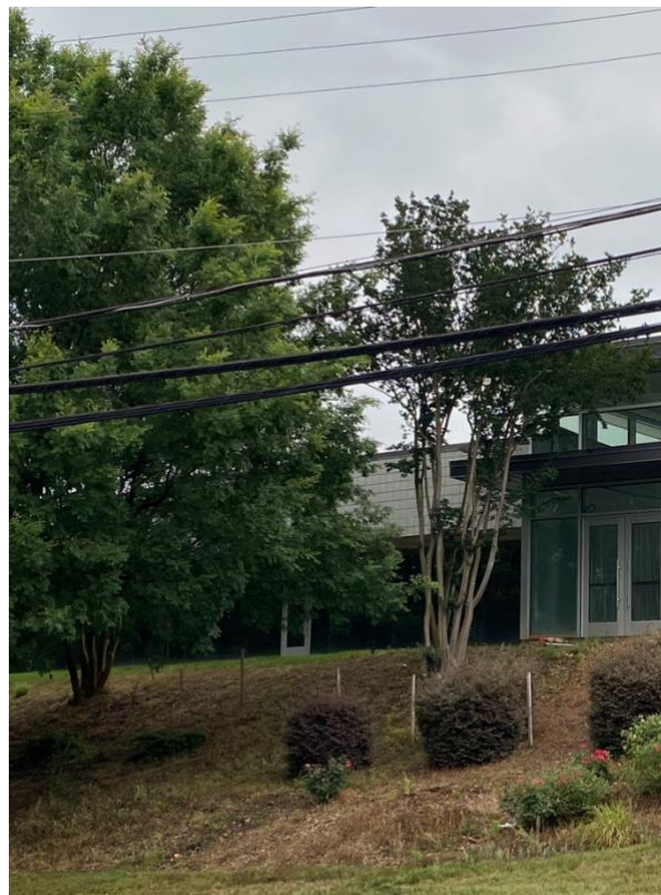
Trees and Landscaping Must Coexist with Utility Lines in the Right-of-Way.
