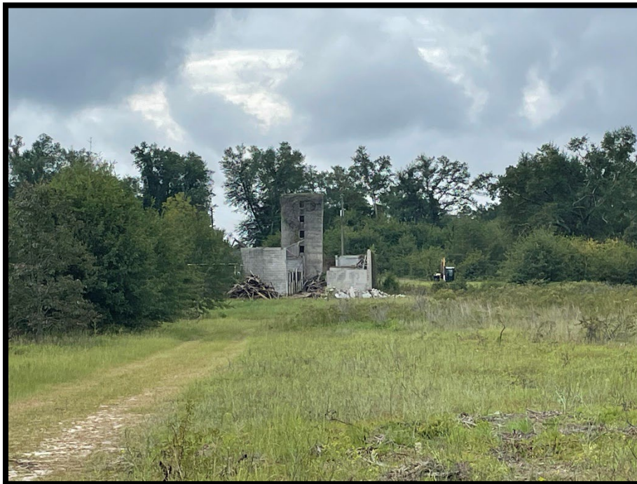
Abandoned Structure on Parcel
