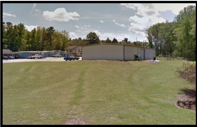
Looking south across Alpha Rd.
