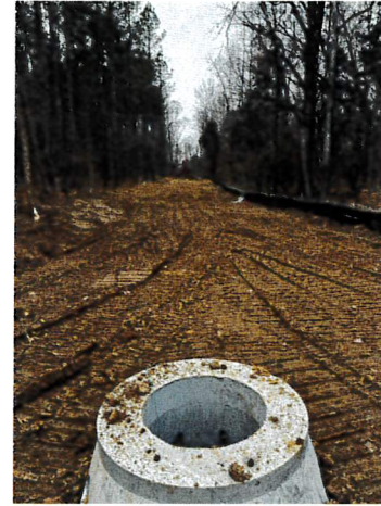
Sewer Trunk Line under construction
