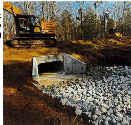
Activity Road Culvert
