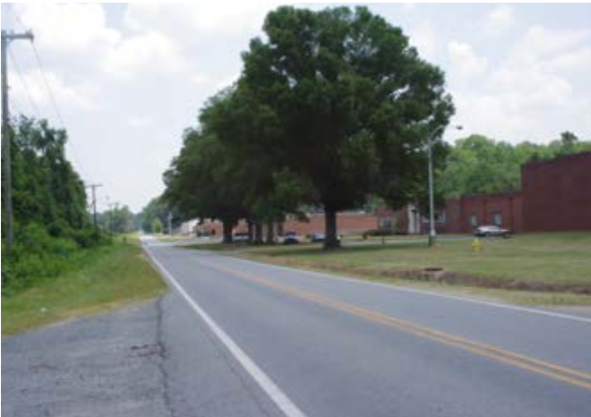
Light Industrial Center
