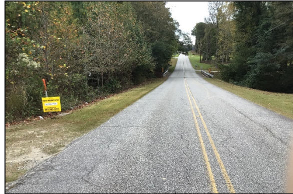
Looking north along Pineview Drive with subject parcel on left
