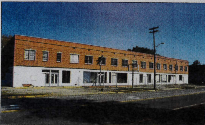
This is the current state of the Ellen Dean Hotel building.
